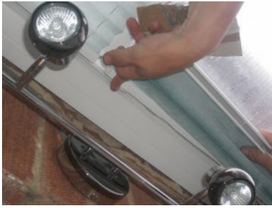
FIX THE BOTTOM RAIL INTO POSITION
