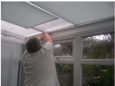
FIX THE TOP RAIL IN POSITION (UNDER TENSION)
